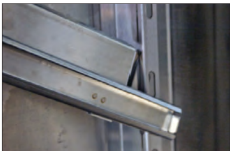
Fig. 9: Set Rail in New Position
